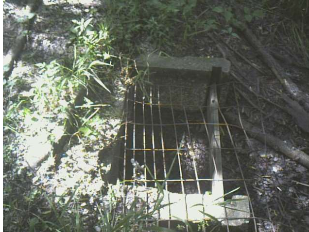
Photo 5 Concrete stop log headwall structure with metal mesh and wood boards in place
