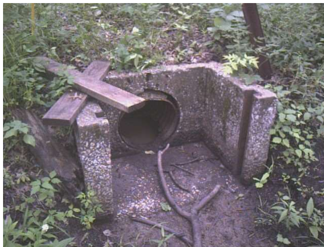
Photo 4 Concrete stop log headwall structure
