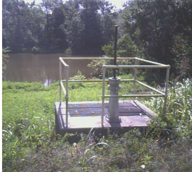
Photo 13 Concrete gatewell on the adjacent Levee
