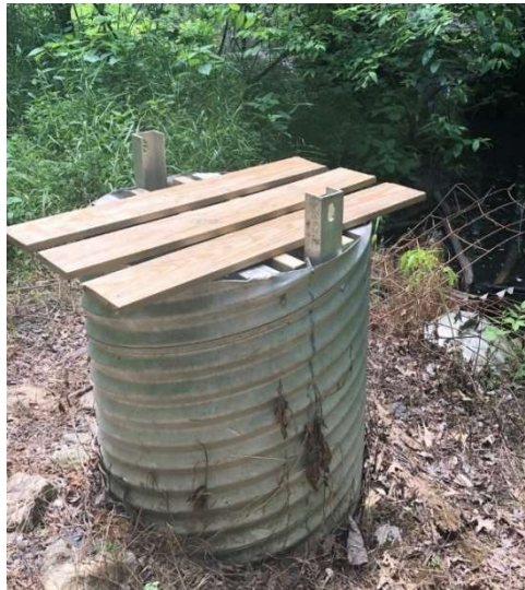
Photo 1 Stop log risers with wood planks cap
