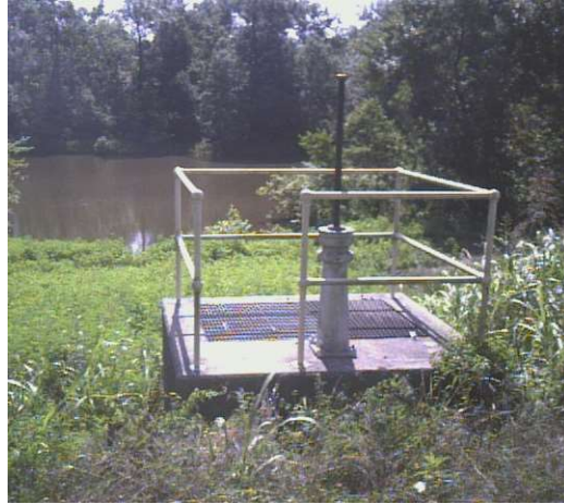
Photo 27 Example of metal grating on top of gatewell structure
