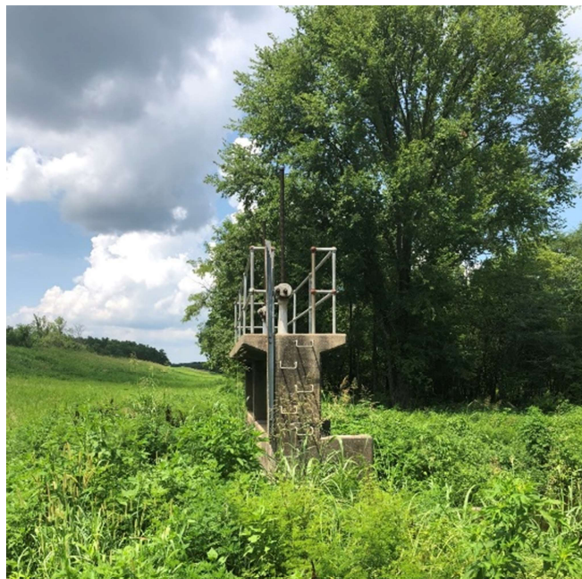
Photo 14 Concrete headwall structure on the Grand Tower Levee
