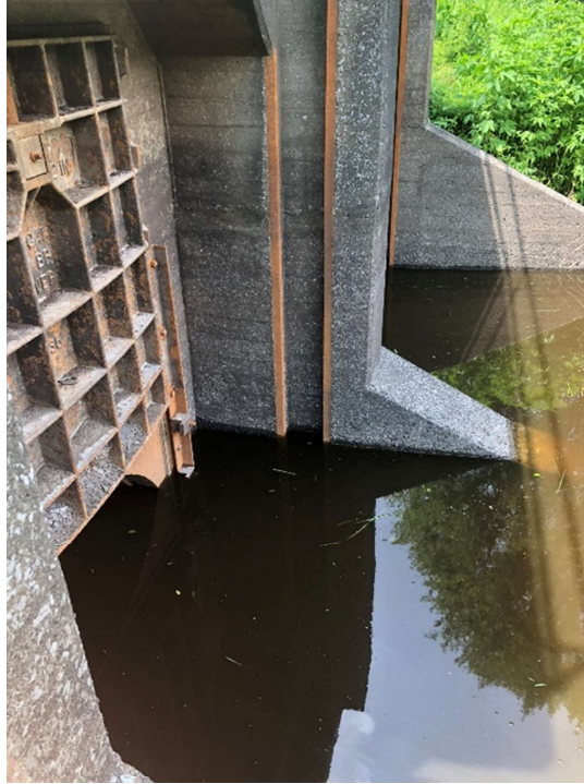
Photo 15 Slide gates installed on concrete headwall structure on the existing adjacent levee
