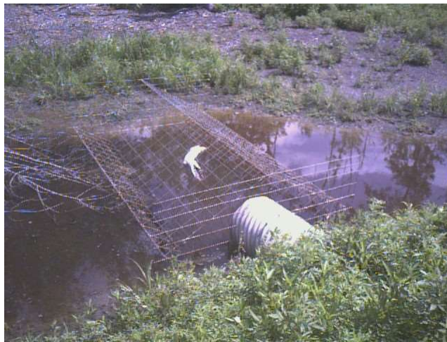
Photo 6 Open corrugated metal pipe culvert with mesh guard box
