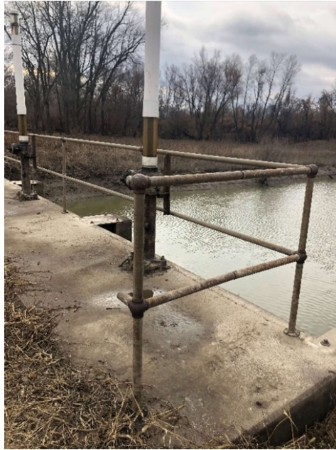
Photo 25 Typical guardrail on headwall structure
