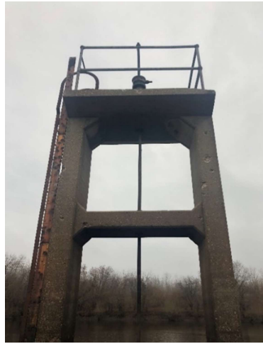
Photo 24 Slide gate installed on reinforced concrete headwall structure
