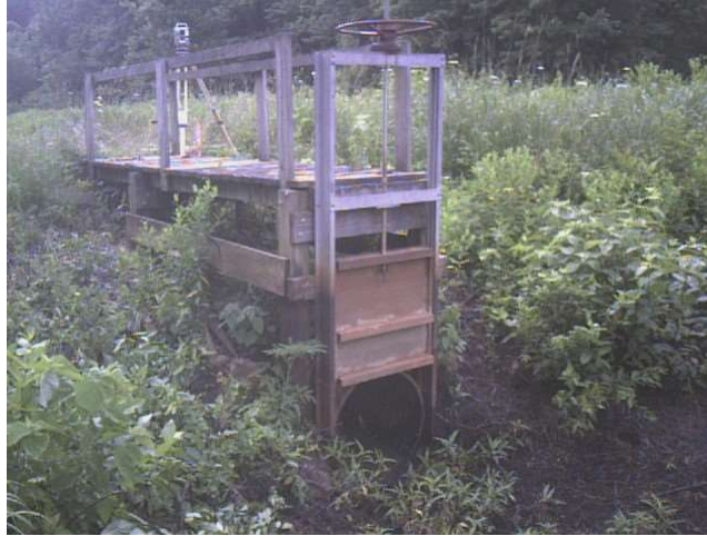
Photo 8 Walkway bridge access to slide gate control structure
