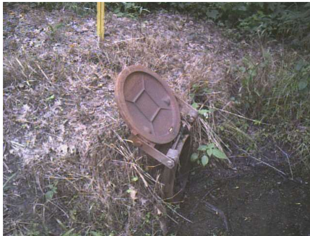
Photo 12 Fully-open flap gate showing underside of leaf
