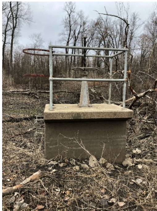
Photo 26 Typical guardrail and rungs on headwall structure
