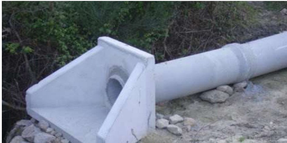
Photo 18 RCP and headwall/wingwall assembly during construction
